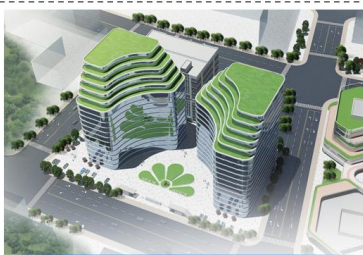
Optosky Technology Park (Xiamen North Station) – Under Construction
