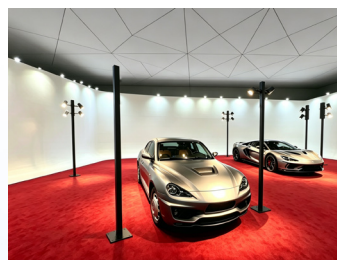
Exhibition hall lighting
