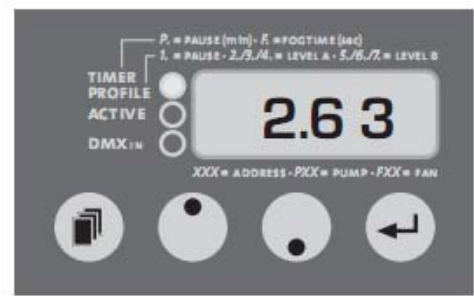
Fig. 7: Adjusting the pump
