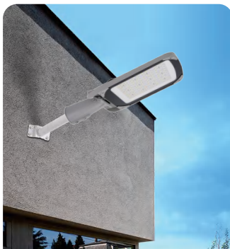
Wall straight rod installation
