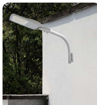
Wall bend installation
