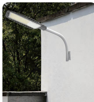
Wall bend installation
