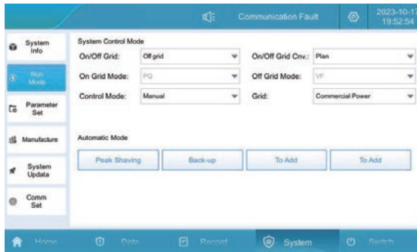
Figure 5.20 Manual and off-grid switching mode setting interface
